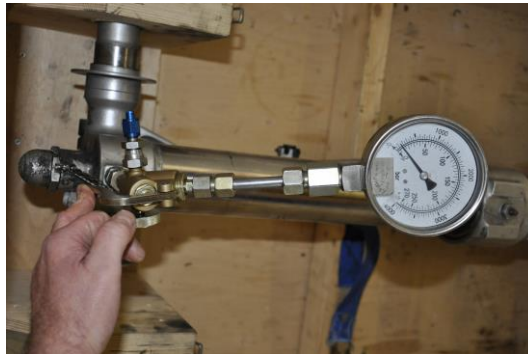
Photo 10: nitrogen pressure measurement.
