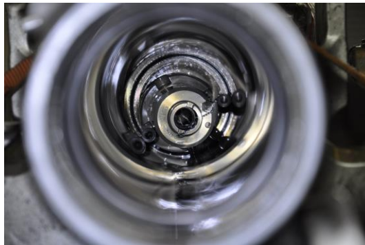
Photo 13: visual observation of the valve housing, piston and locking cylinders (dowels).
